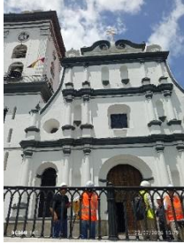
a) Fachada Principal
