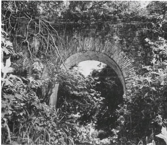
Figure 57. Section of an old colonial aqueduct in the Aragua Valleys, which may have inspired Dr. Caudri to paint one of her paintings showing this type of hydraulic work. Source: ARCILA (1961)
